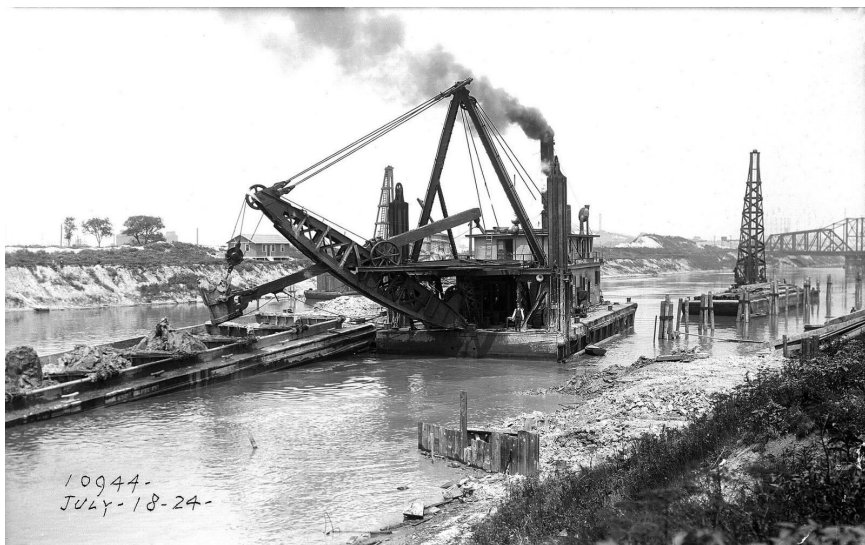
Dredging a cofferdam on the Sanitary and Ship Canal at Cicero Avenue, 1924.
