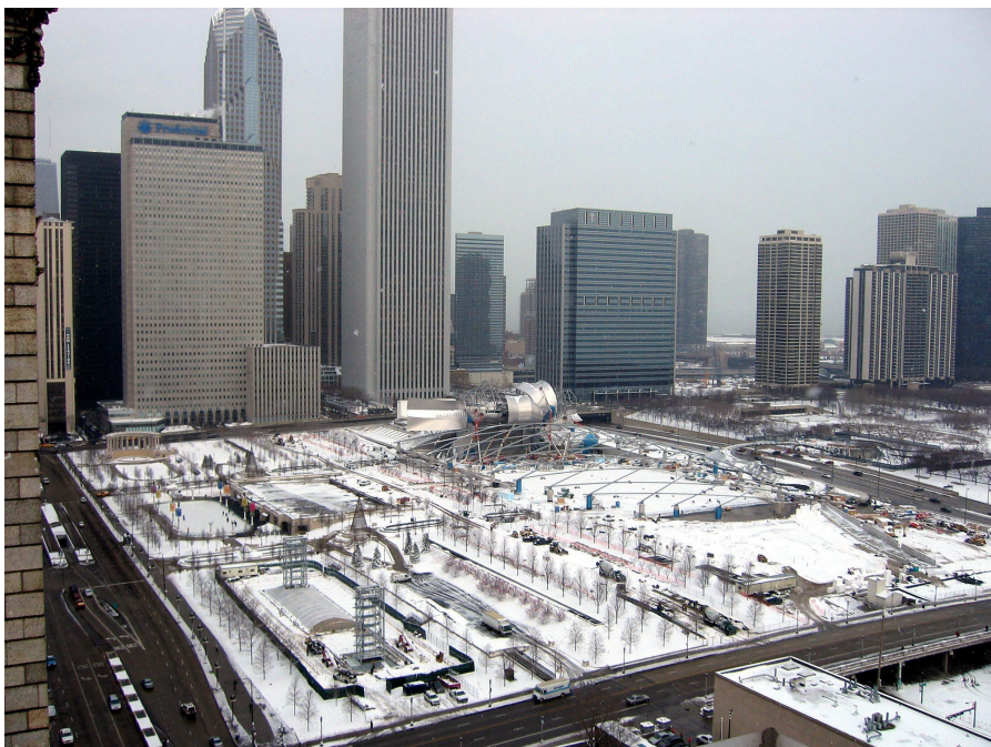
January 5, 2004 view from The Cliff Dwellers of Millennium Park under construction after a snowfall.
