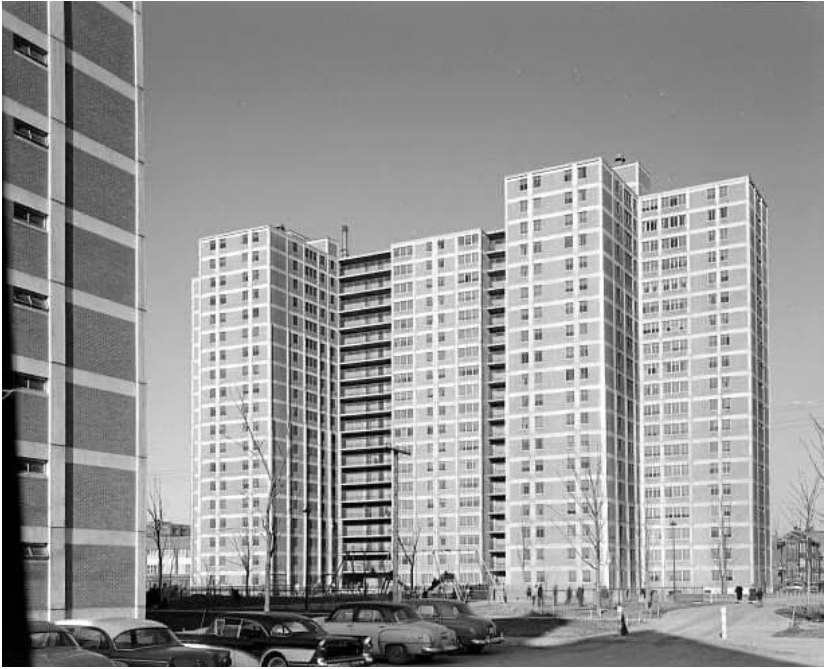
High-rise towers at Cabrini-Green, Division and Larrabee Streets, 1958.
