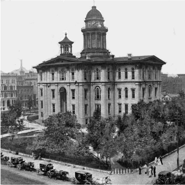
The Court House and City Hall after the city raised its street grade — a fourth floor was added in 1858 to match the new elevation.
