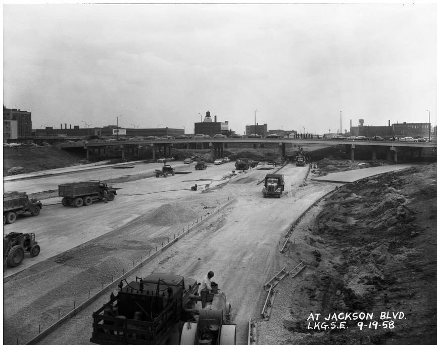
The Kennedy Expressway at Jackson Boulevard, under construction, 1958.
