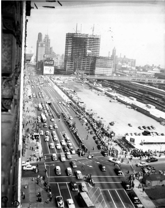
View from the Auditorium Building to the Prudential Building under construction, 1954.
