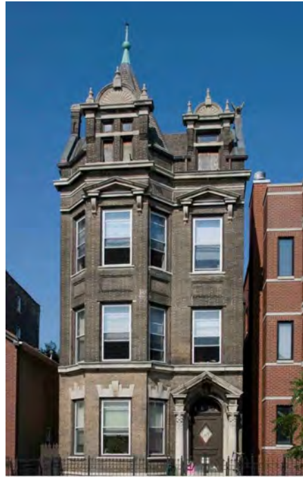
2010 1852 South Allport Avenue. The Pilsen neighborhood is a living museum of 19th century vernacular architecture
