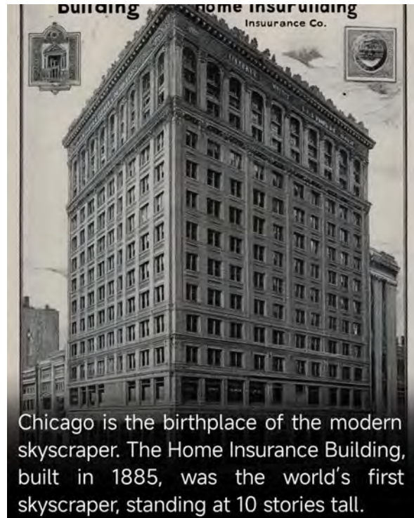
The Home Insurance Building, 135 South LaSalle Street, 1885 — conventionally credited as the world's first skyscraper.
