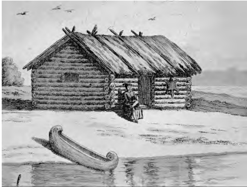
The west bank of the Chicago River's north branch, near Wolf Point — site of Jean Baptiste Point du Sable's log cabin, where he farmed and traded.
