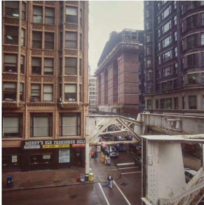
The Harold Washington Library under construction, 1991, named for the mayor who broke the machine's grip on Black political loyalty.
