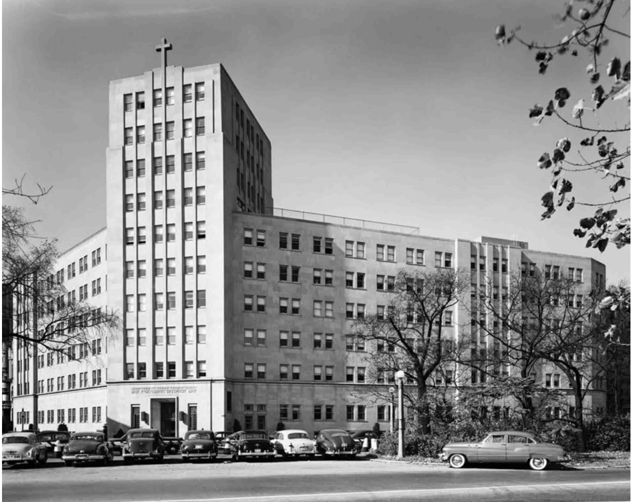
1950 Columbus Memorial Hospital, 2520 Lakeview Avenue. View west from Lincoln Park.
