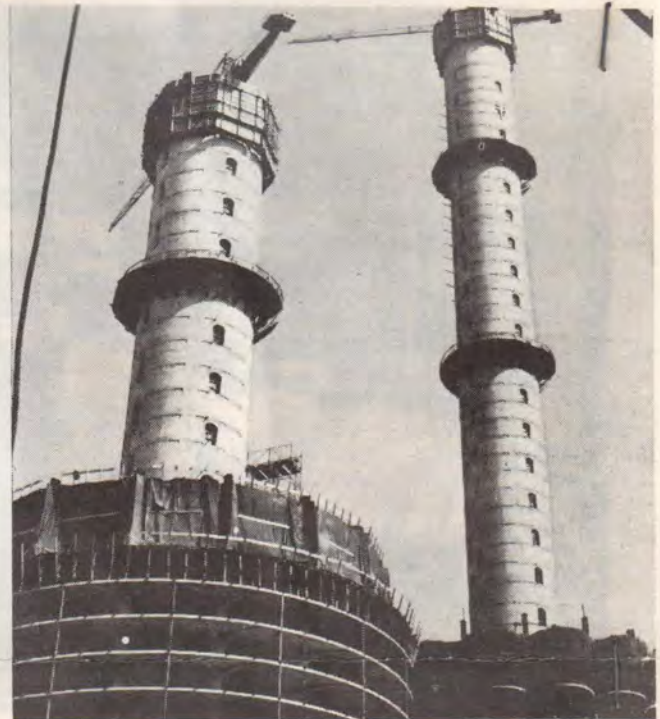
Center service cores are completed a long time ahead of the surrounding floors, permitting early start and completion of all service facilities. A Linden crane is at top of each core.
