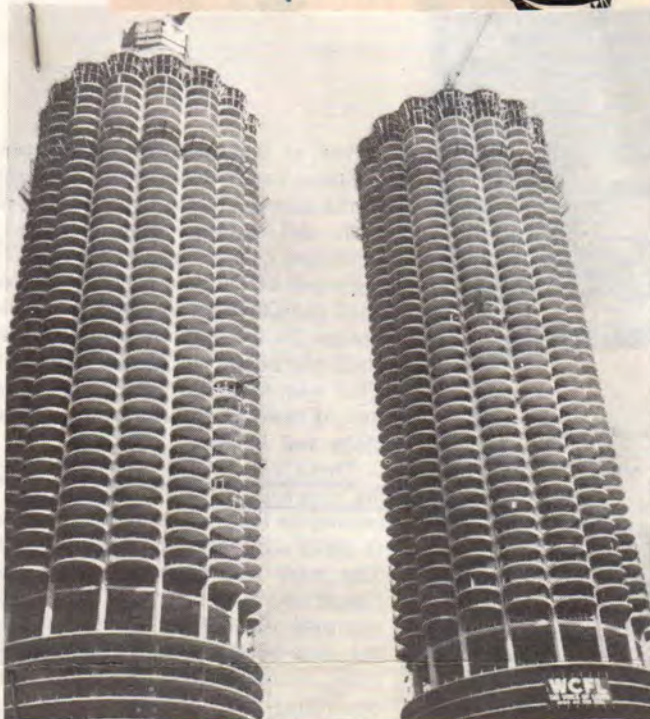
Construction of round apartment towers nears completion. East Tower (right) is at top apartment floor (60th), West Tower at 57th floor. Note separate balcony for every living room and bedroom.
